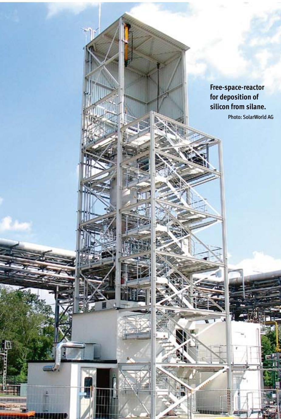
Free-space-reactor for deposition of silicon from silane.
